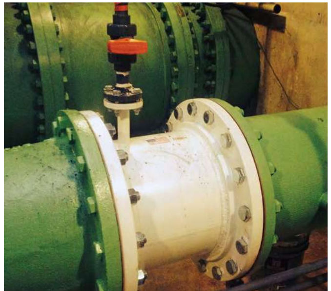
UltraTab mixing alum into water at a Colorado municipality
