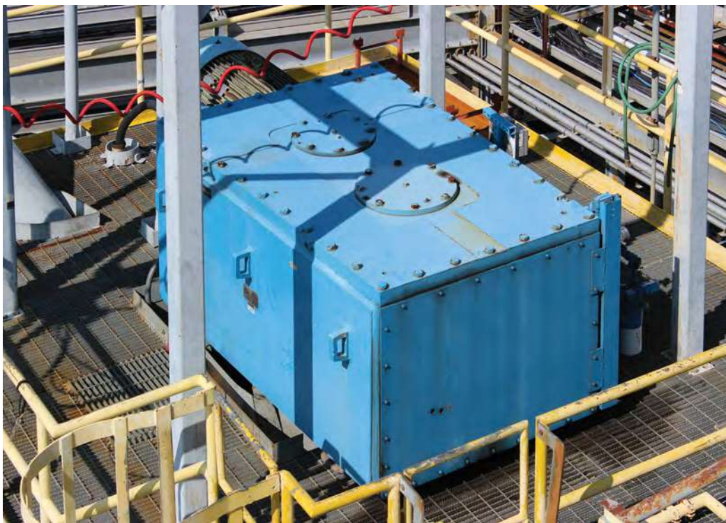
Installed Chemineer HT agitator
