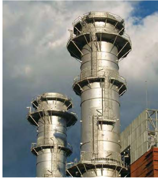
Exhaust stacks at a power plant in the Midwest
