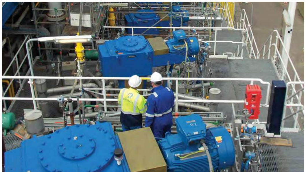
Field service technicians are readily available to help maintain your equipment as shown in this large chemical plant in the UK
