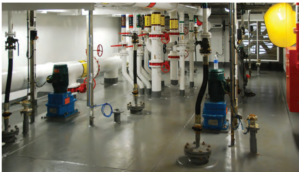
Installed Model 20 agitators on an oil rig
