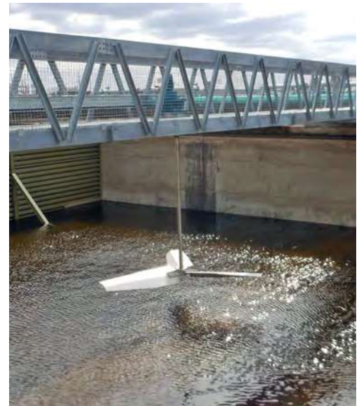
Installed XE-3 impeller at a wastewater treatment facility
