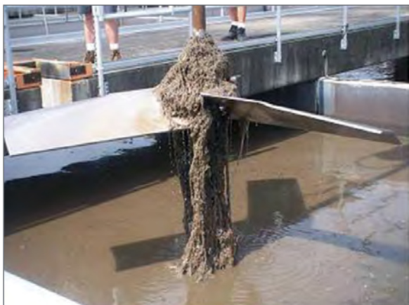
HE-3 impeller ragging after eight weeks in operation at a Florida wastewater treatment facility
