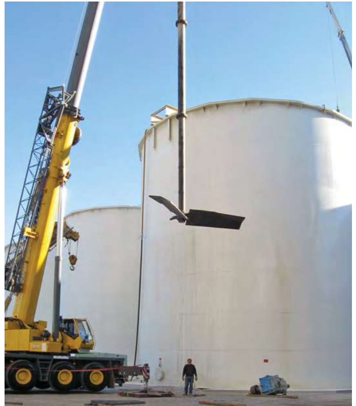
Field service technicians can assist your crew or handle the complete installation for you
