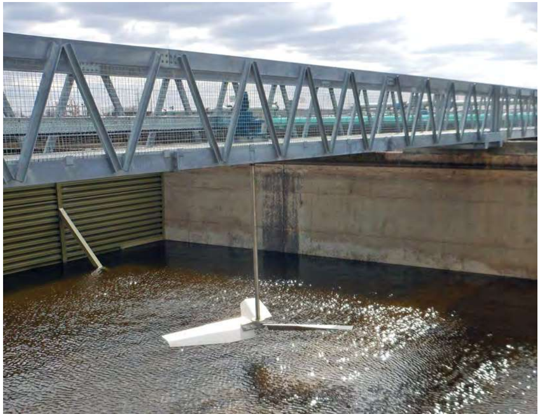
XE-3 impeller installed in a wastewater treatment facility in the United Kingdom
