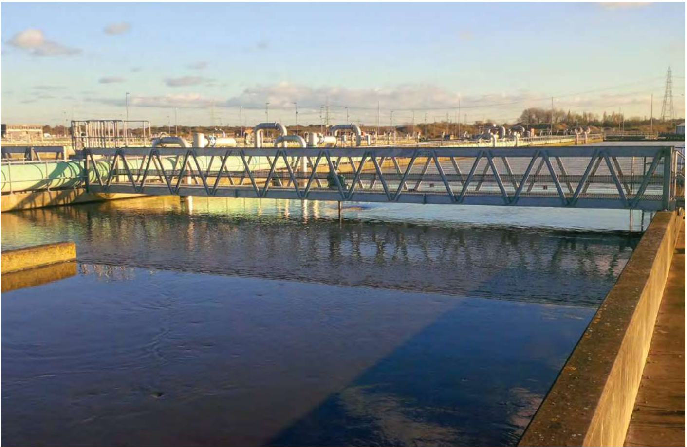
One of twenty-four Chemineer agitators installed at this facility for water treatment
