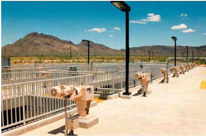
HT agitators working to treat waste and suspend solids at an Arizona treatment facility
